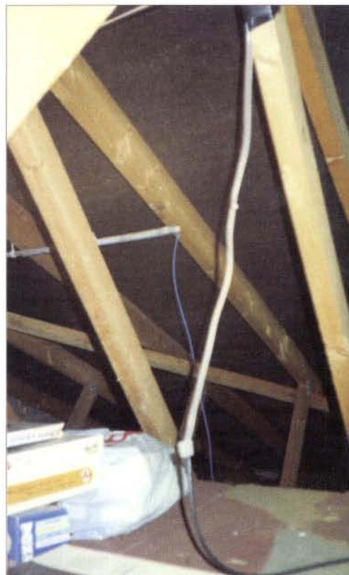
Fig. 3: With the dipole elements taped to the beams in the loftspace, the feed line can drop vertically down, free of any other object in the loft (see text for photograph information).
